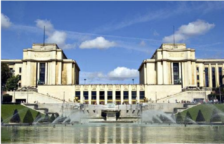
Figure 1. Palais de Chaillot (Paris, 1937), made of concrete with supersulfated cement.
